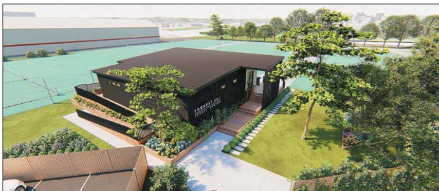
New look...an artist's impression of what the new building will look like.
